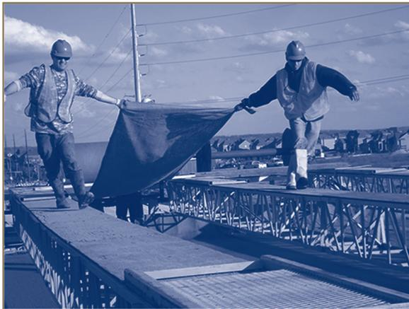
Figure 1. Pre-cut, rolled, wet burlap is placed within 10 minutes of strike-off.
